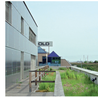
Photo-voltaic facade at SOL4 building, Mödling
